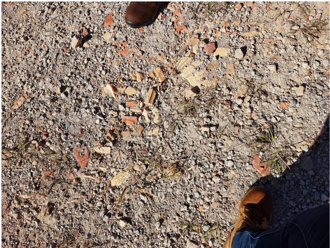
Photograph 4 - Fill material including bricks in access road on western entry to site
